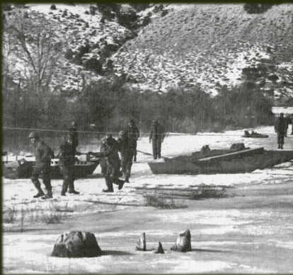
Members of the 1457th Engineer Battalion, 19th Special Forces Group, 163rd Armored Cavalry Regiment, and 140th Field Artillery assisted in channel clearing, water supply protection, roadway repair and dike construction in Utah County.
